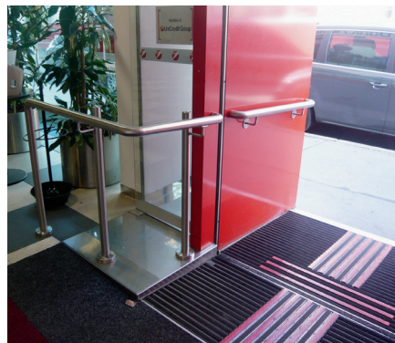
Accessibility in many forms: there are no steps at the entrance and a tactile guiding system leads from the entrance area to the information desk.
